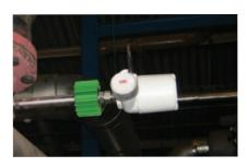
The ABB transmitter is powered by an on-board micro-thermoelectric generator (micro-TEG), driven by the temperature difference between the steam pipe and its surroundings.
